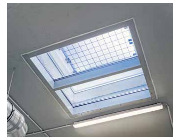
Weather protection due to light dome
